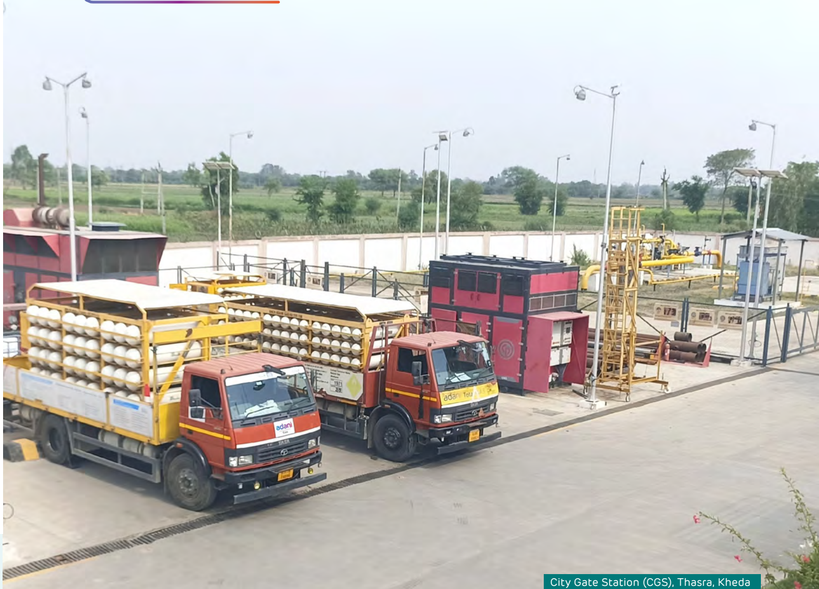
City Gate Station (CGS), Thasra, Kheda
