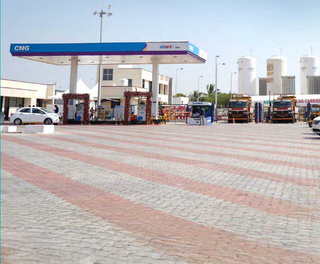
Liquefied Compressed Natural Gas Station (L-CNG), Tiruppur
