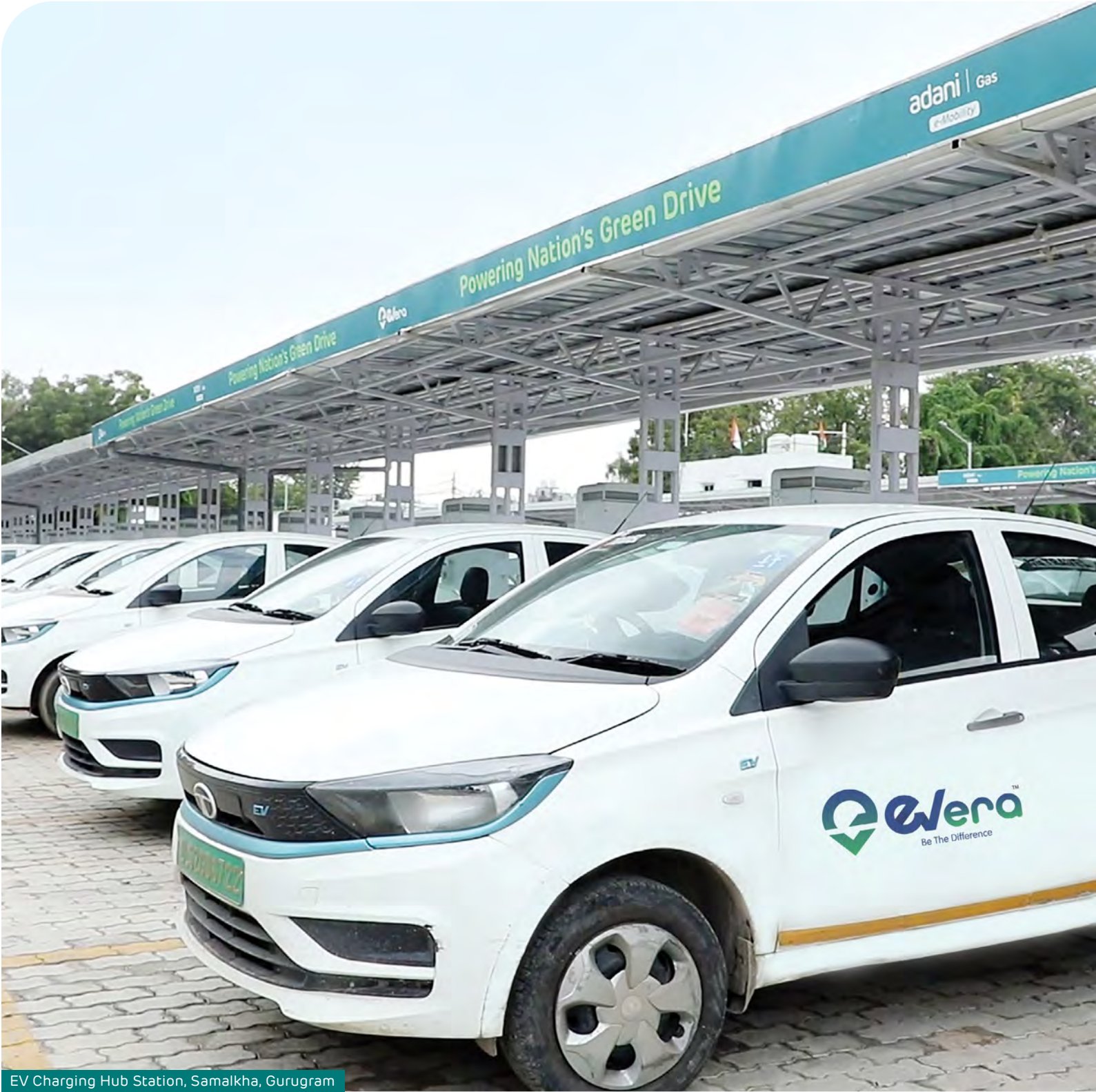
EV Charging Hub Station, Samalkha, Gurugram
