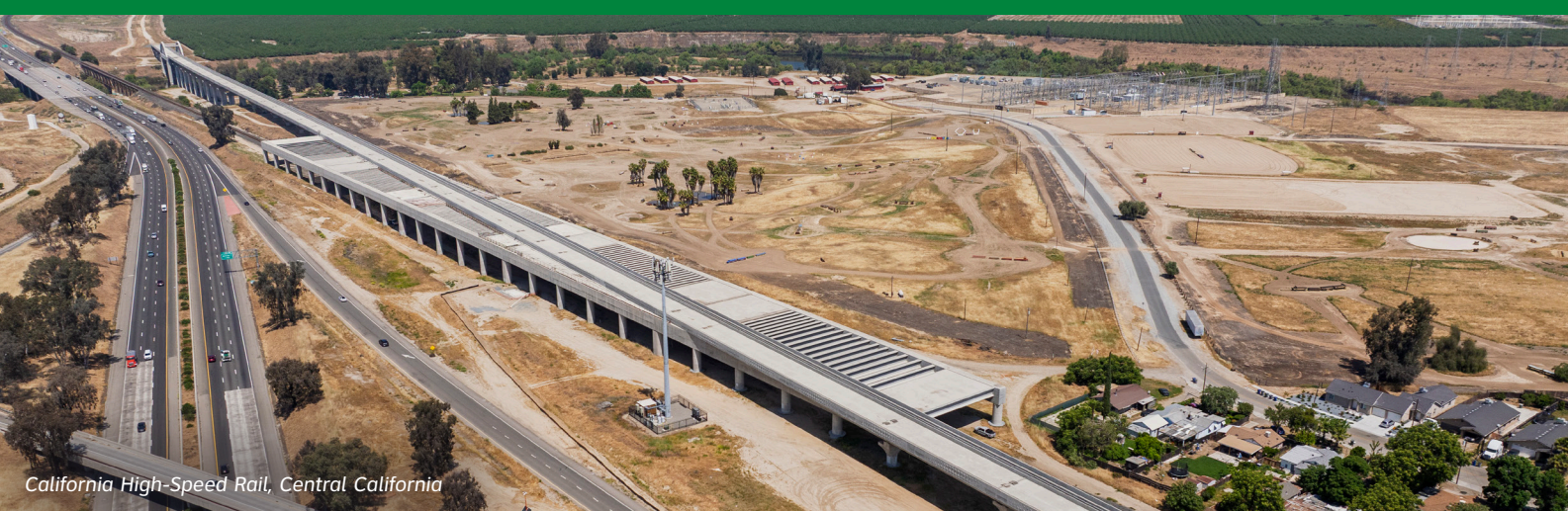
Purple Line Extension, Los Angeles, CA
